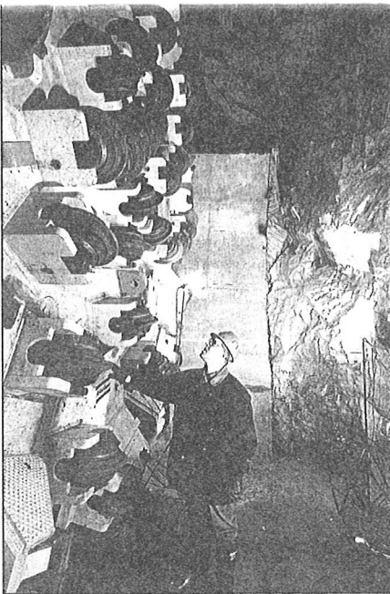
Cutterhead on the Markham/Atlas Copco Robbins TBM for the NYC water tunnel.
